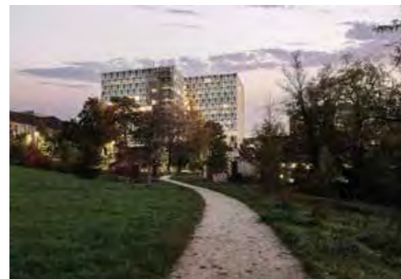
Construction area 12: The new main building Anna-Seiler-Haus is now visible by its illumination and the "Insel"-letterings on its roof.
