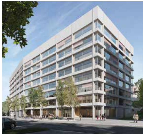
Panel 7: The front of project "JANUS", the future building of the medical research and training center (©ARGE BB07)
