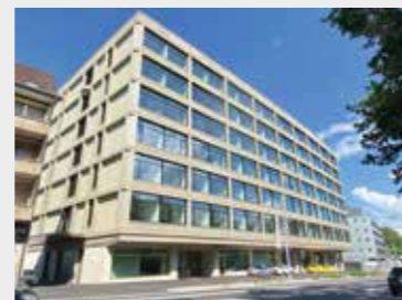
Front view Murtenstrasse 24-28
