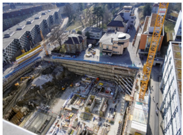
Construction place panel 12.
