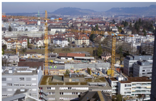
The construction site of the Murtenstrasse 24.
