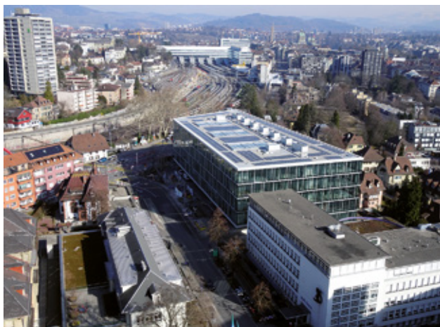
View from the top of the Bettenhochhaus towards the Railway Station. At the front right the school of dental medicine, in the center the new building of sitem-insel.
