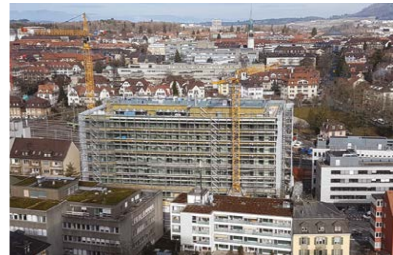
Murtenstrasse 24-28 The new modern laboratory building for the Faculty of Medicine is being constructed
